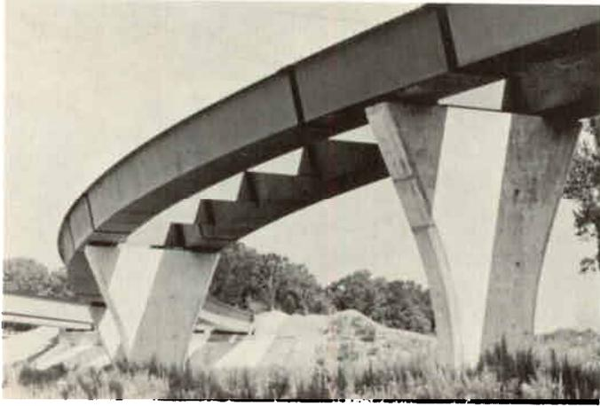
**Figure 65** Louisiana Airline Highway Interchange: erected curved-box girders.
