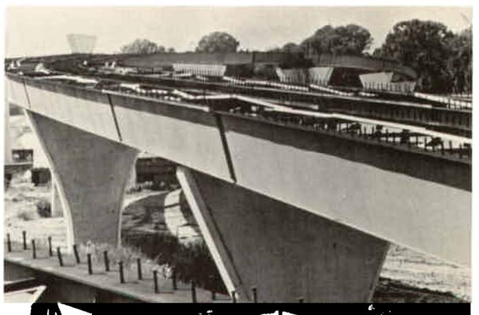
**Figure 64** Louisiana Airline Highway Interchange: erected steelwork.
