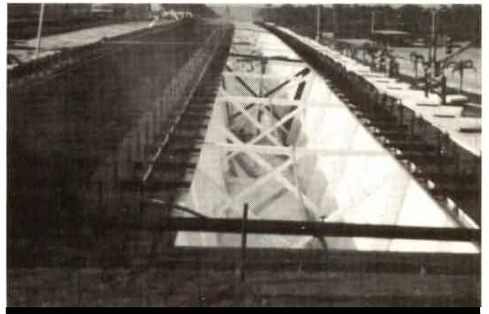
**Figure 80** Bowing of Girder.
