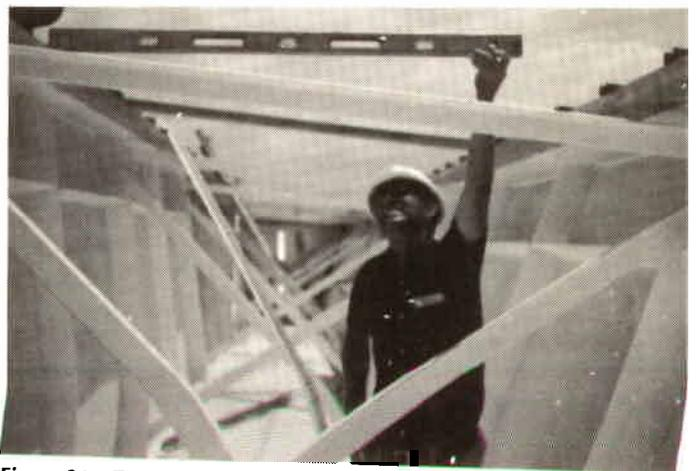
**Figure 81** Twist of Girder.
